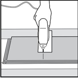
4. If cutting with any power saw, the laminate surface should be turned down. If cutting with a handsaw, the laminate surface should be face up.
